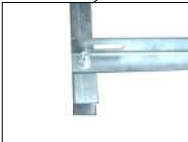
Place the L shape supporter as in photo. Notice that the oval hole is used to support the collector
